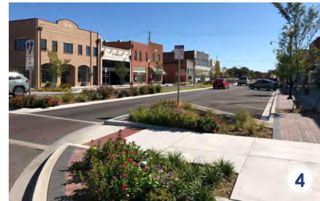
4 Provide landscaping and bulb-outs in parking areas to enhance pedestrian safety and experience
