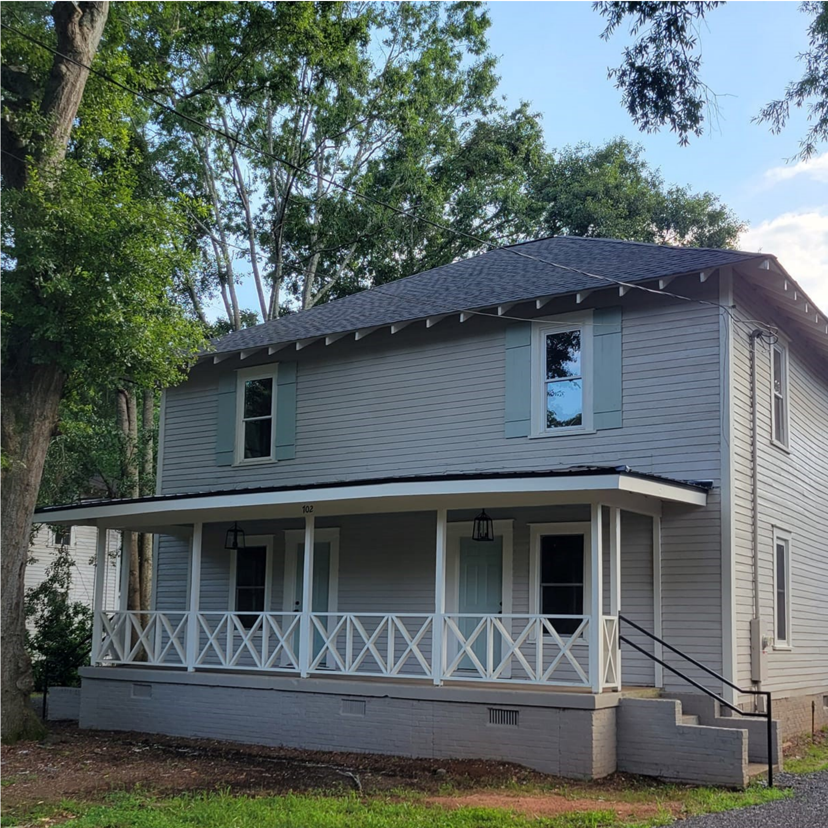
3 - 2-story structure at 702 Radford Street
