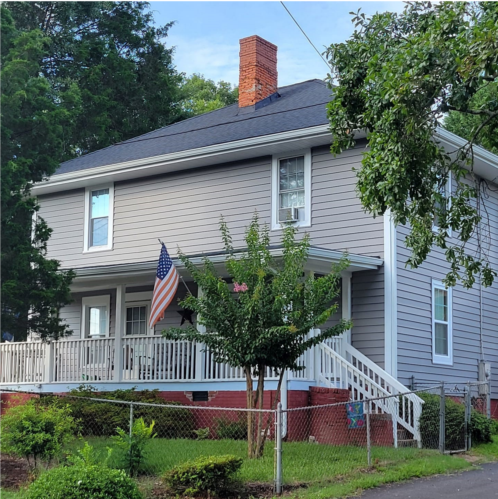
2 - 2-story structure at 705 S. Madison Ave
