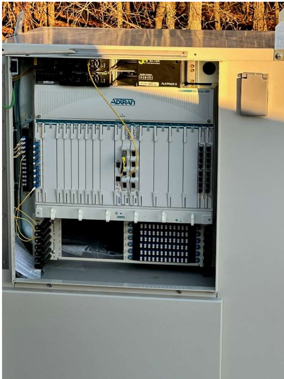
Our new fiber OLT which has been configured, installed, and is getting ready for service deployment.
