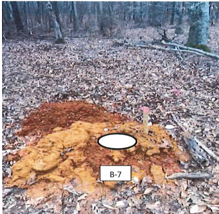
Location of Boring B-7 (Approximate Station 3+29±); Looking West
