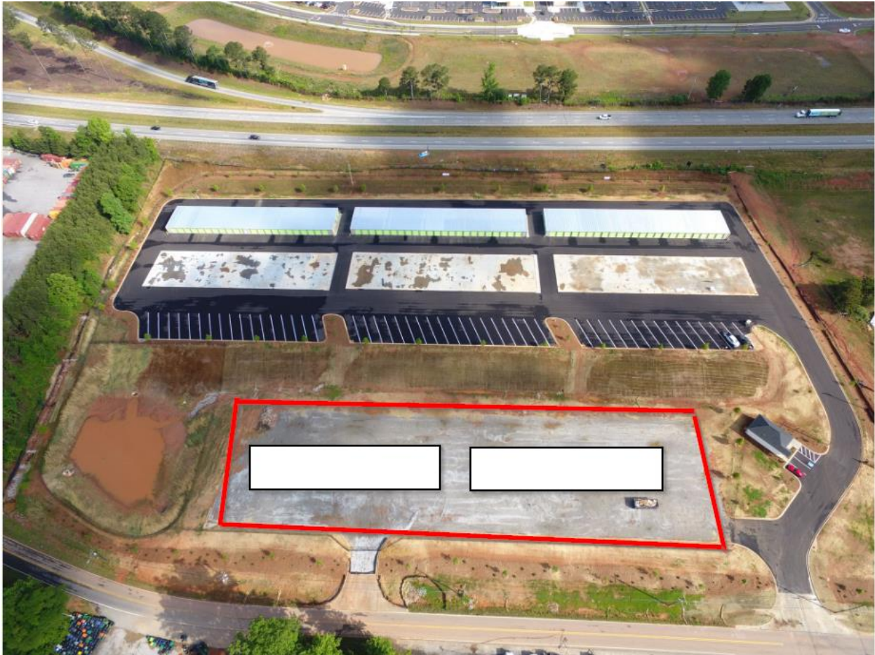
Aerial image showing buildings 7 and 8:
