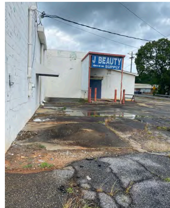
View of Rear Side of Existing Building
