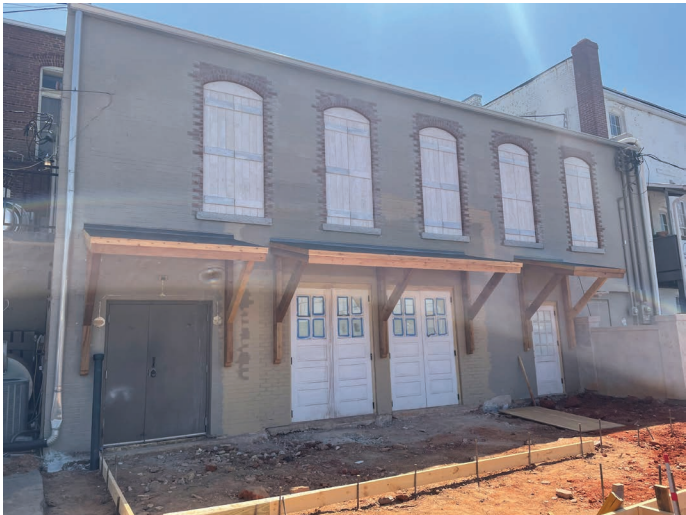
118 North Wayne Street, under construction
