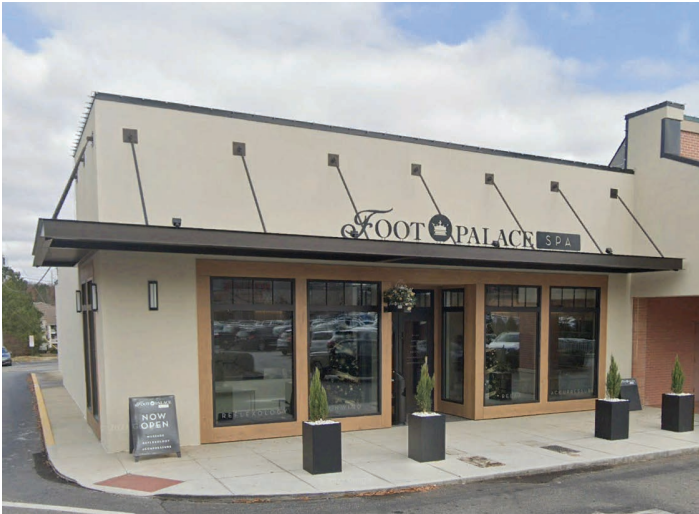
Beechwood Shopping Center, after renovations
