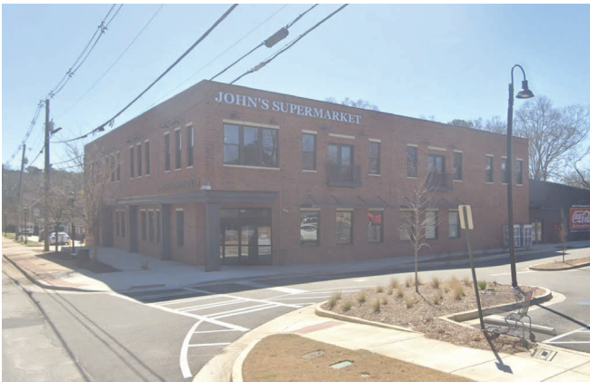
416 South Broad Street, completed project
