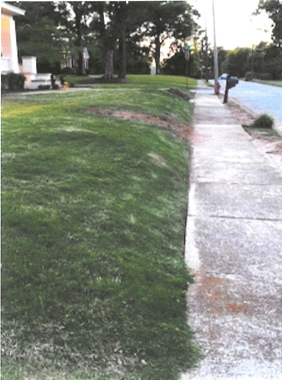
Erosion due to loss of trees that were deceased or dead
