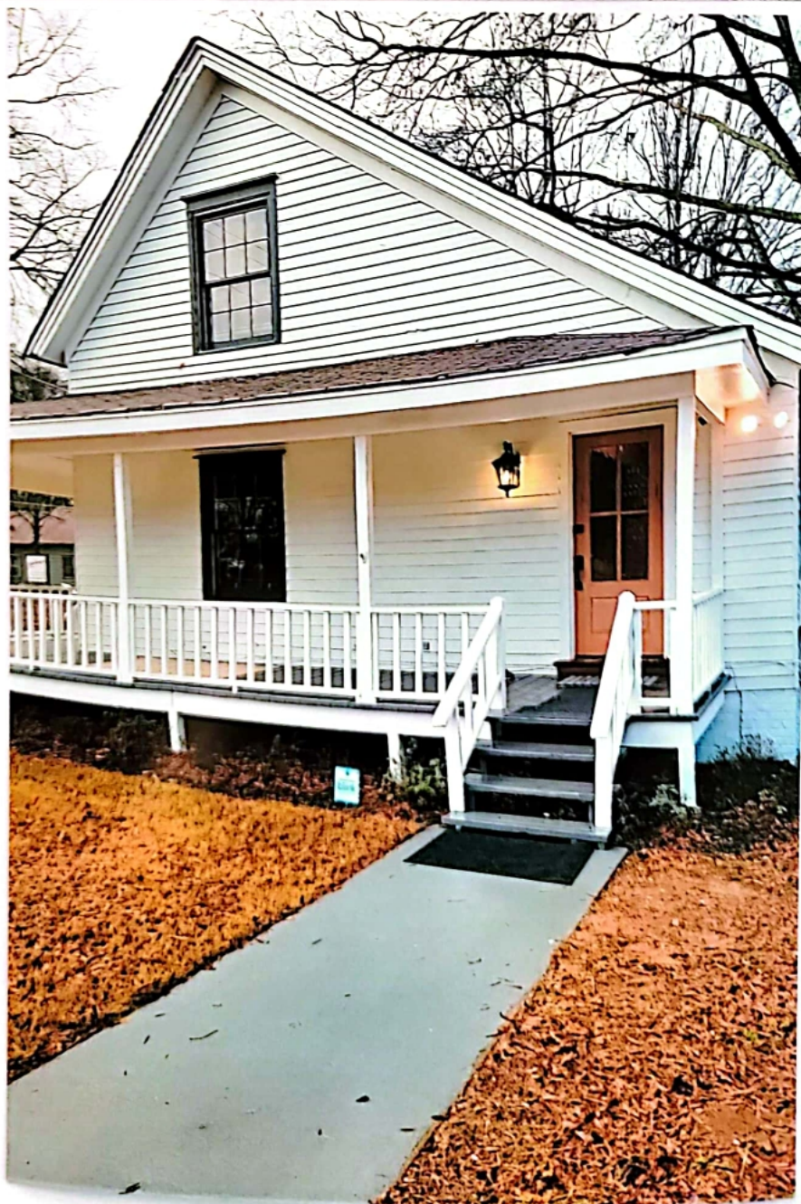
104 3rd St remodel to match style/ colors of the remodel that we completed on 706 S. Broad St in January 2022.
