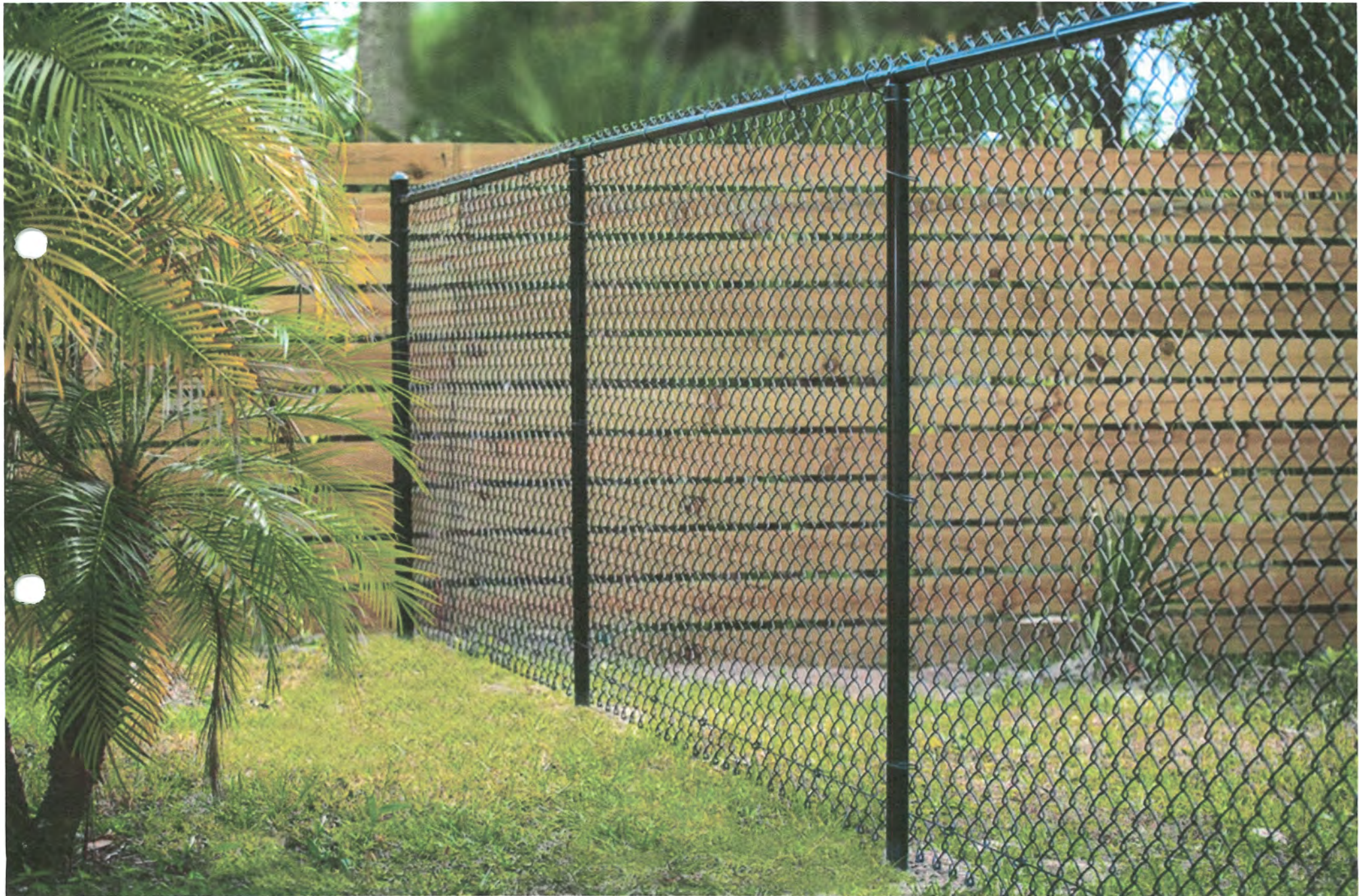
Typical section of black chain link fence adjacent to wood fence
