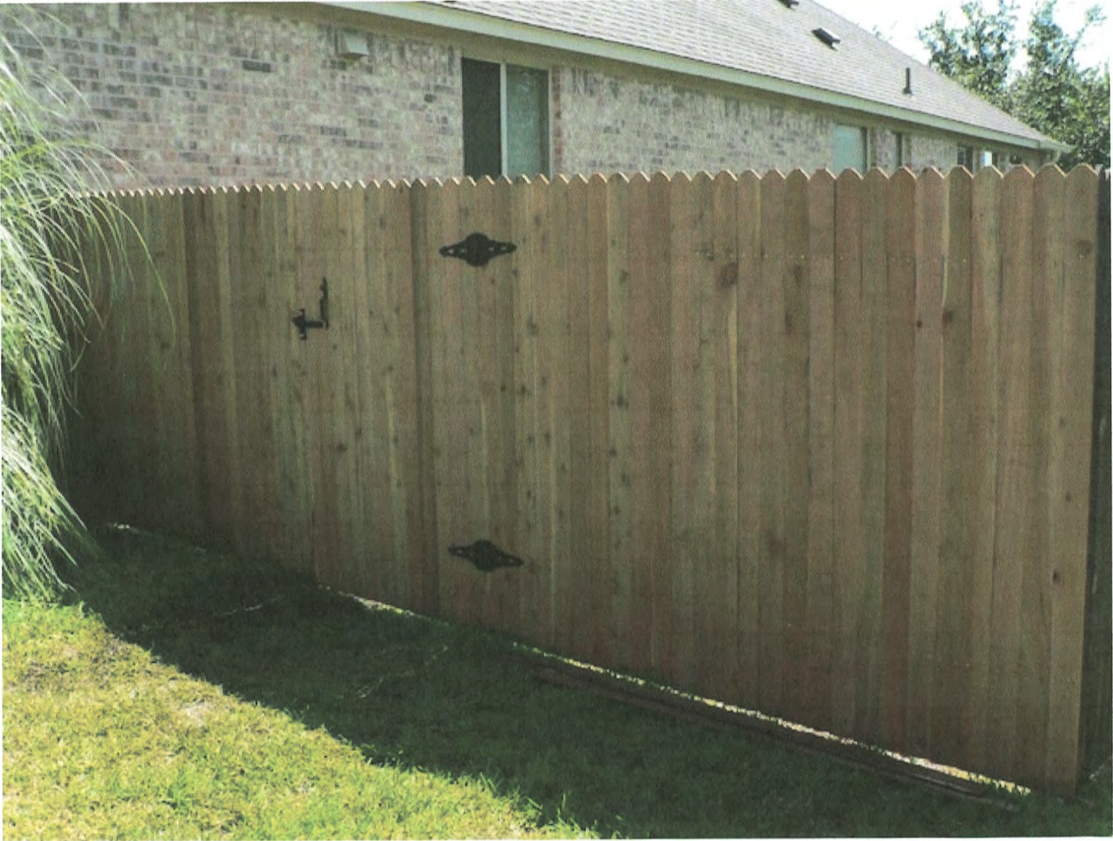
Typical section of wooden fence with gate
