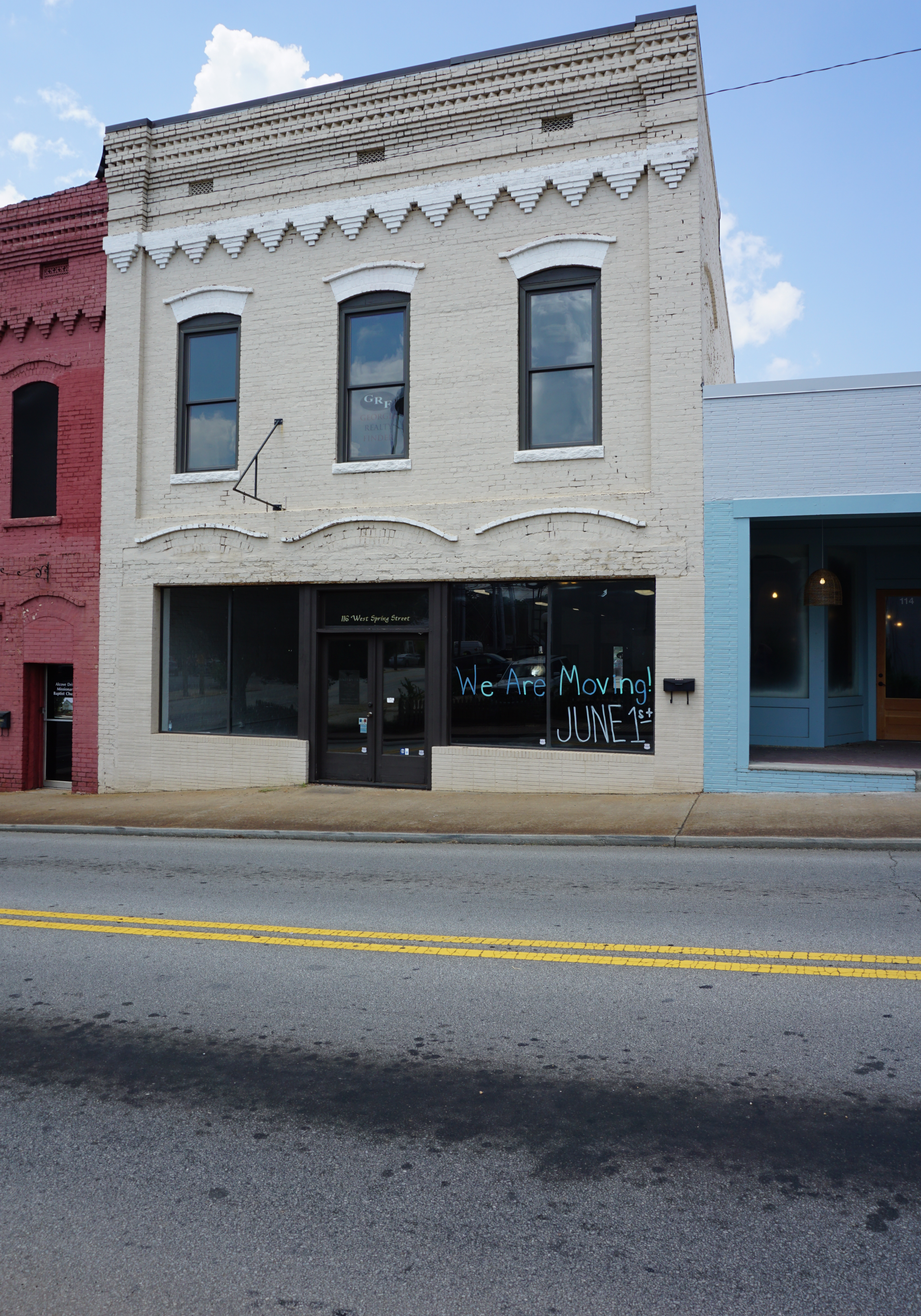
Front facade - Existing Condition
