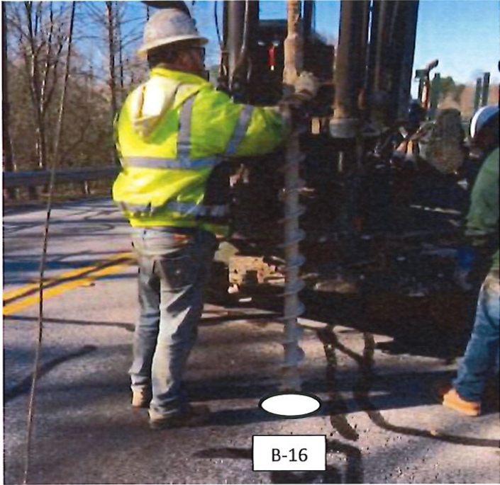
Location of Boring B-16 (Approximate Station 2+75±, 30' RT); Looking West
