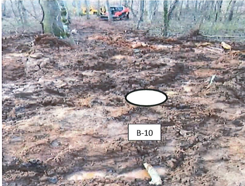
Location of Boring B-10 (Approximate Station 47+00±); Looking North
