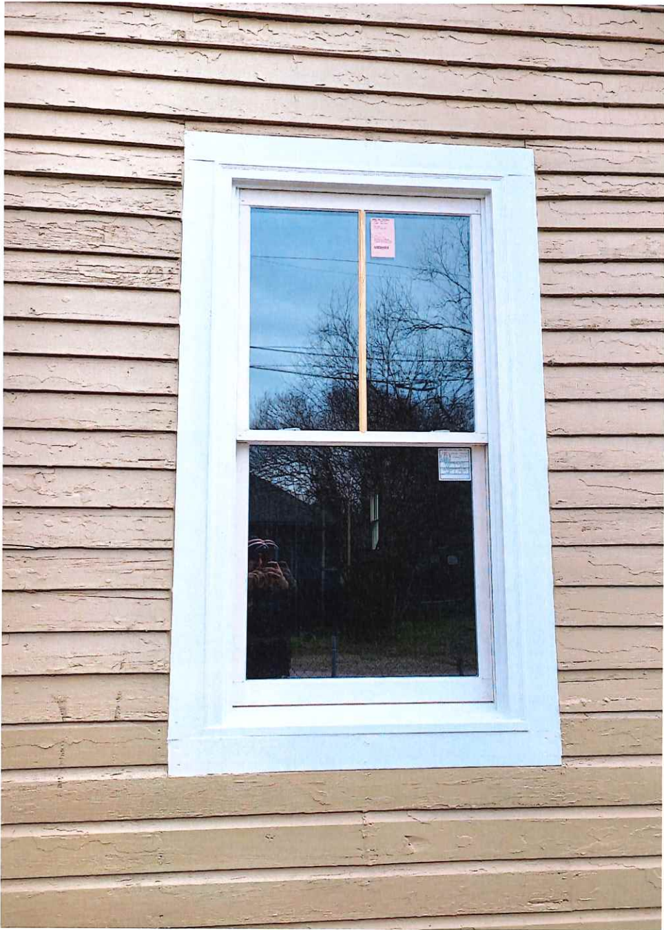
new window sashes
