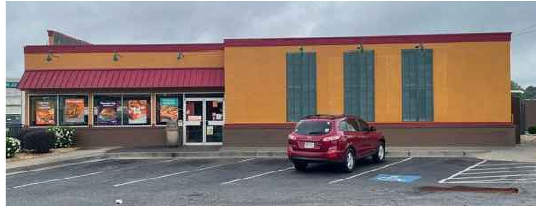
4 EXISTING MAIN ENTRANCE ELVATION A-2.1
