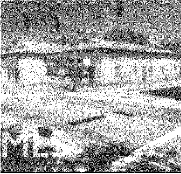
Bldg before Renovation
