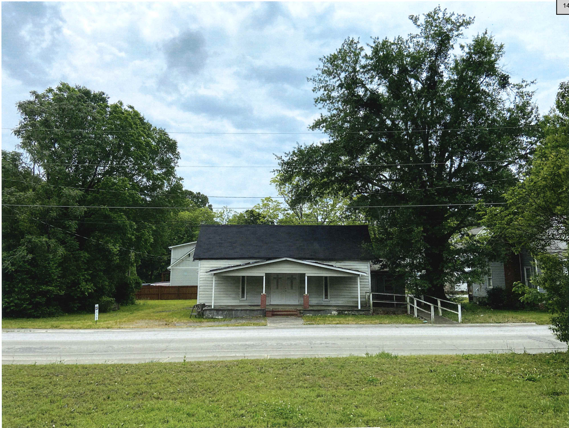
EXISTING STREET VIEW
