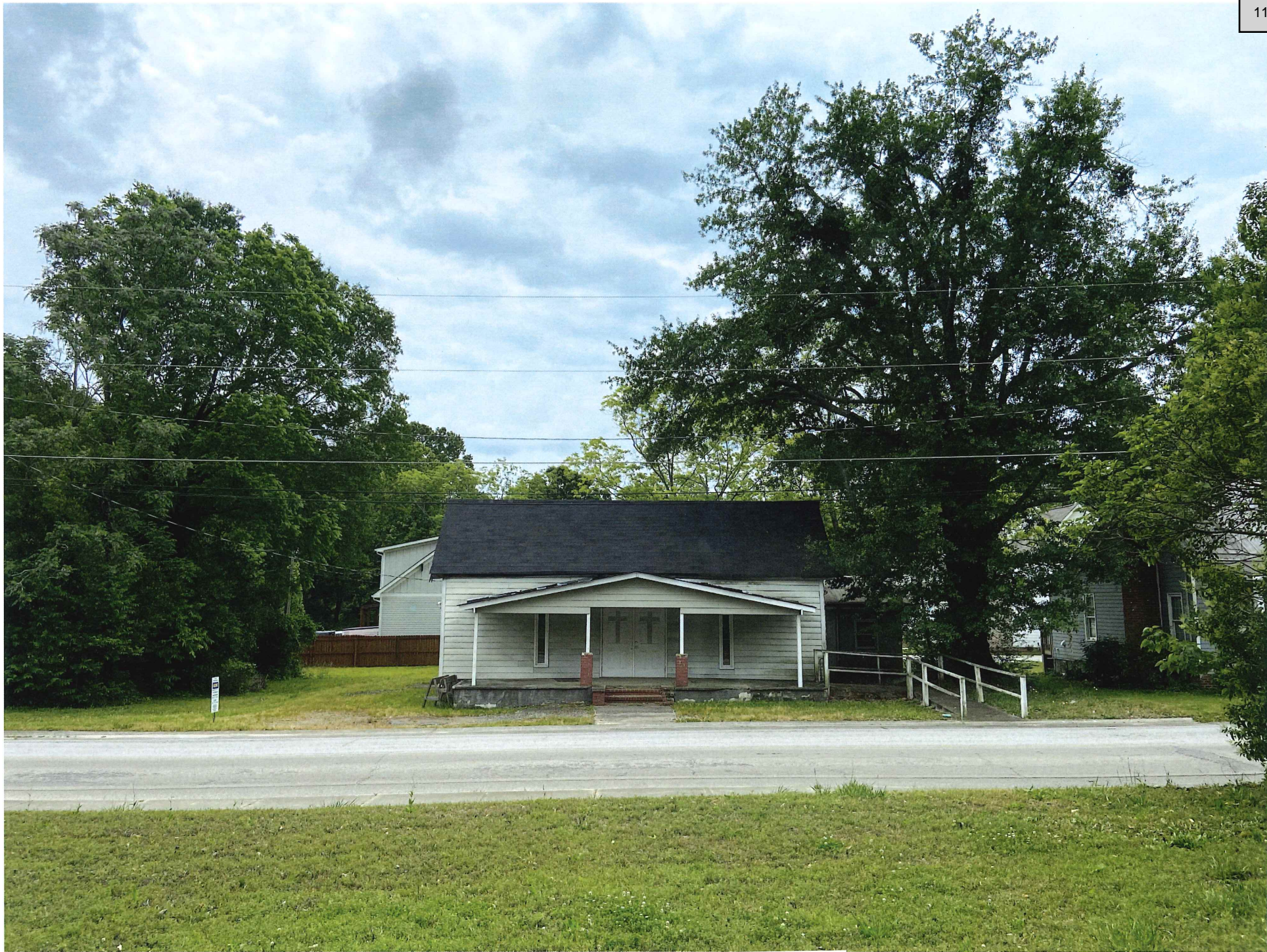
EXISTING STREET VIEW
