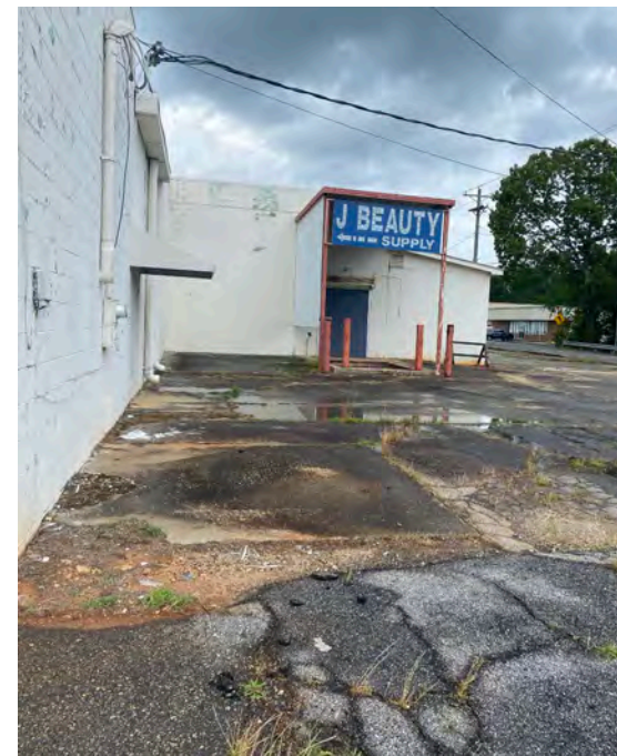
View of Rear Side of Existing Building
