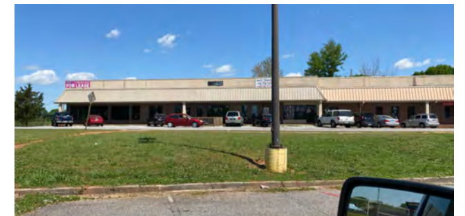
View of Neighboring Development Behind the North End of the Existing Building
