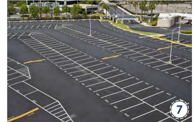
7 Parking lots without landscaping are not permitted. Landscape islands are required
