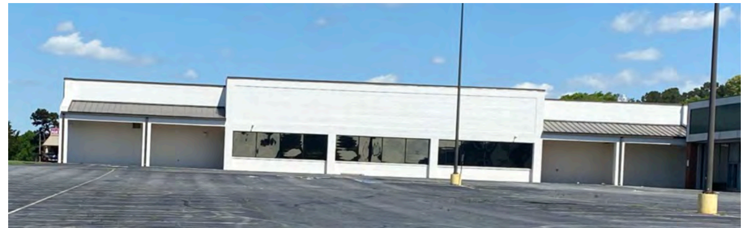
View of Renovated City of Monroe Building
