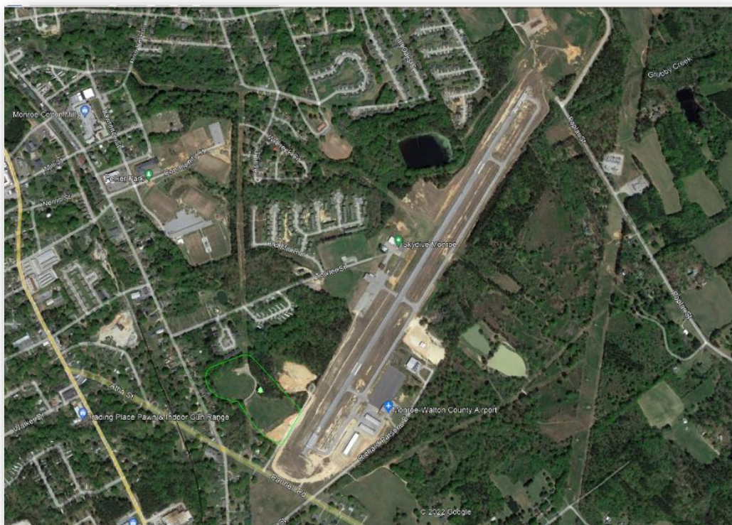
FIGURE 18: AERIAL VIEW OF THE AIRPORT PROPERTY
