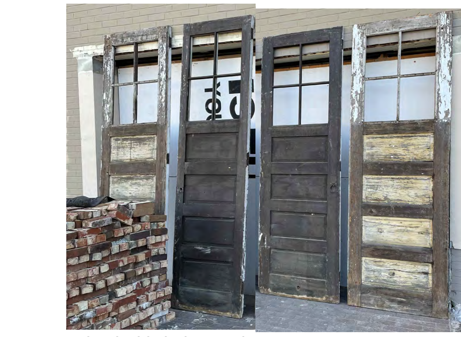
EXISTING DOORS TO BE REUSED
