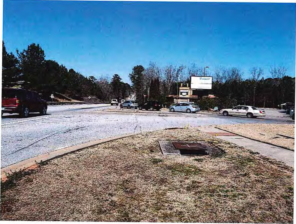
LOOKING NORTH FROM HIGHWAY 138
