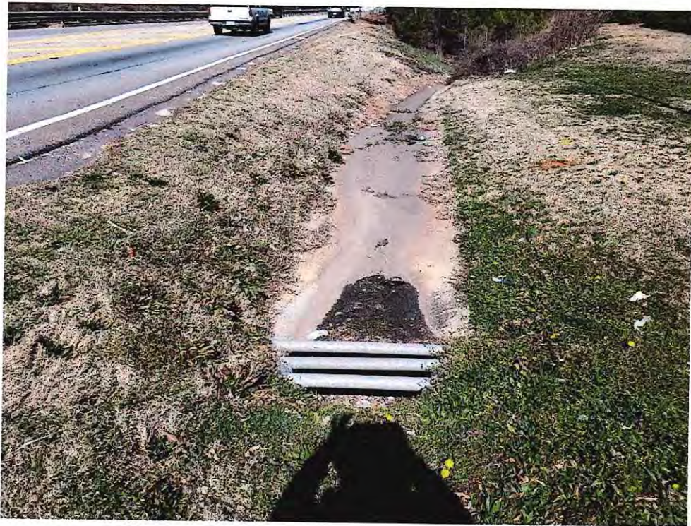
EXISTING DRAINAGE FLUME ALONG HIGHWAY 138
