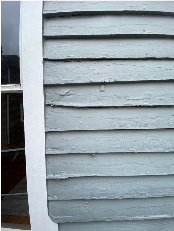
Above is the Southern façade of the structure. This side needs repair with Hardy Board.
