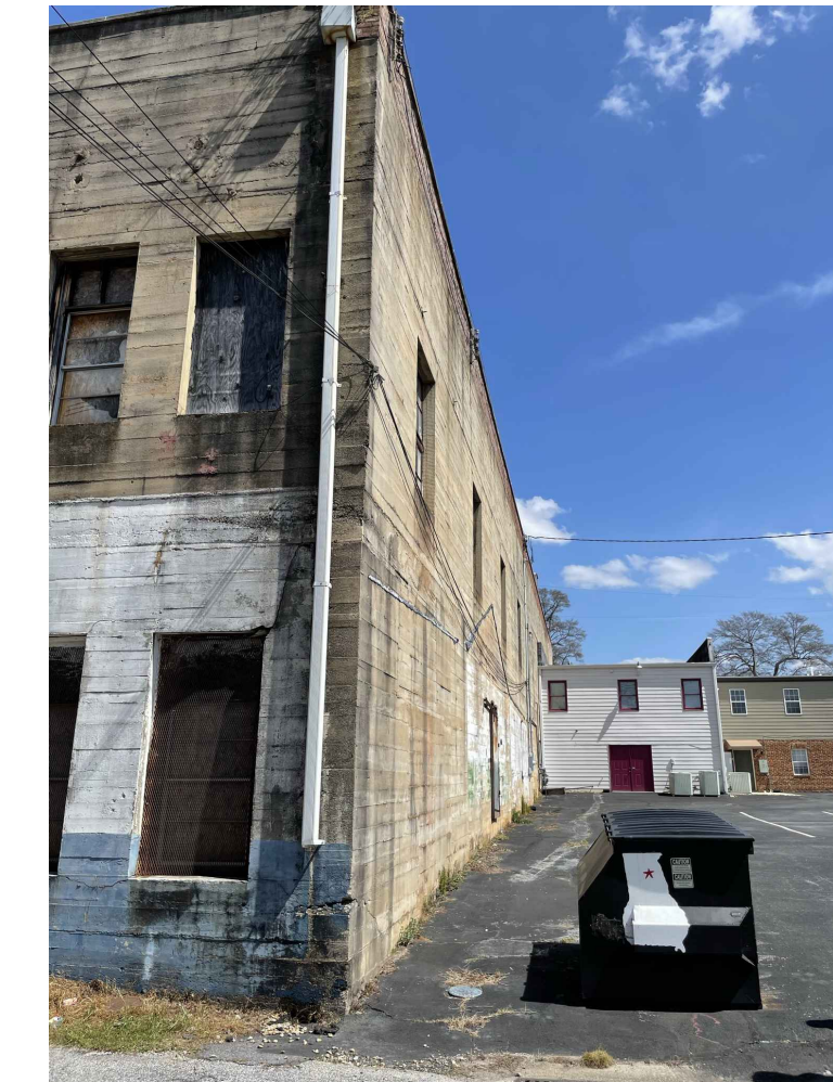
BACK EXTERIOR - FACING N WAYNE ST
