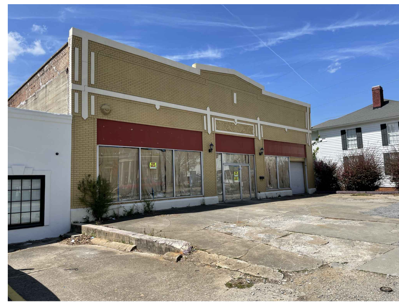
FRONT EXTERIOR - FACING SOUTH BROAD STREET
