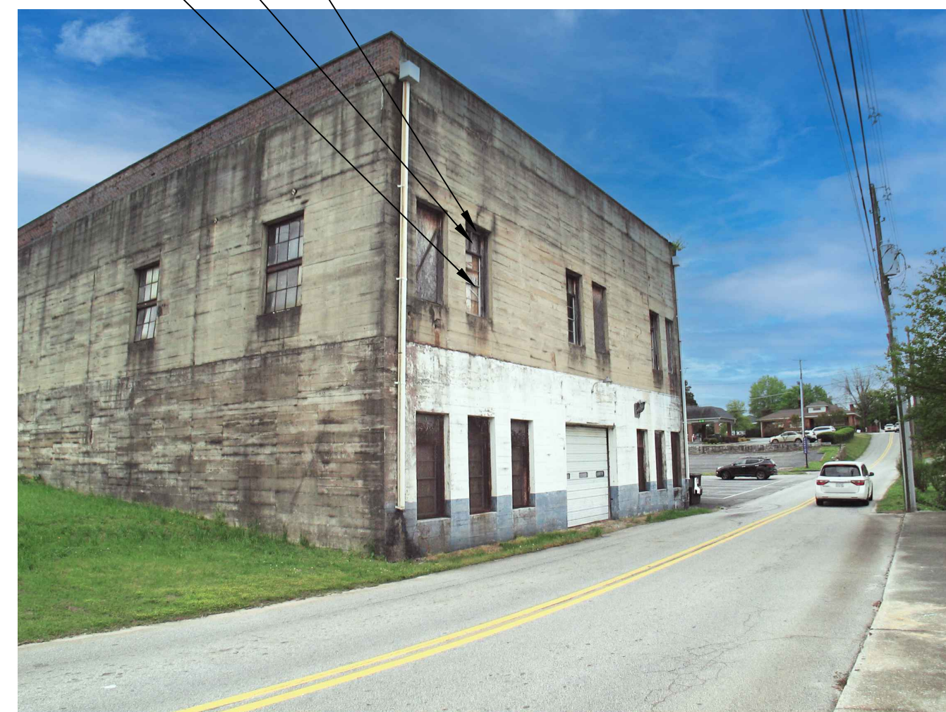
BACK EXTERIOR - FACING N WAYNE ST
