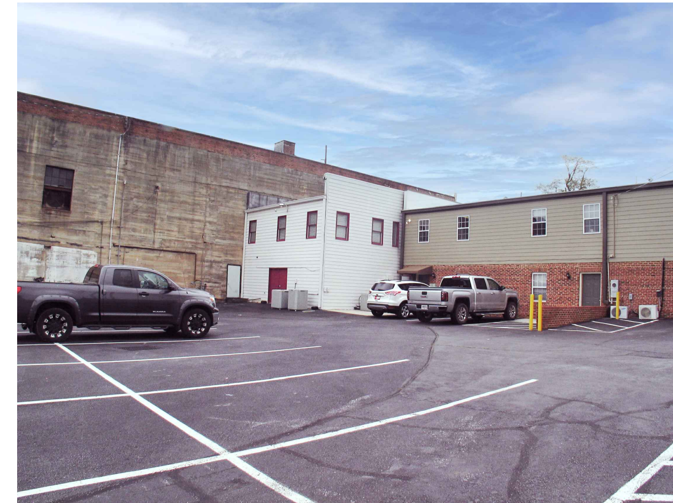
SIDE EXTERIOR - FACING W CHURCH ST
