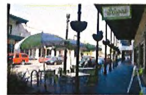
F- Extended second floor balconies
