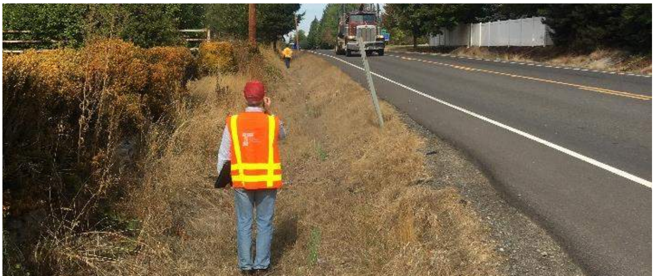
OR 213 narrow shoulder and deep ditch
