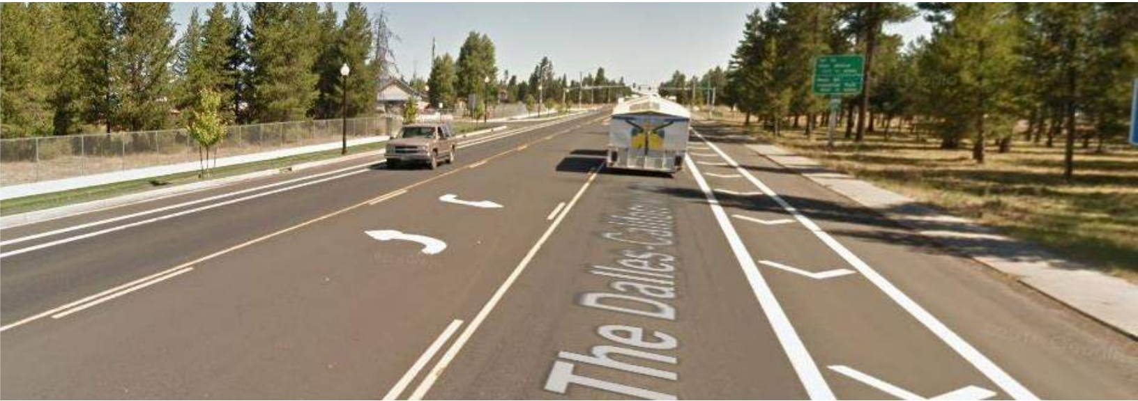
Example cross-section with center two-way left-turn lane, buffered bike lanes, and sidewalks (La Pine, Oregon)
