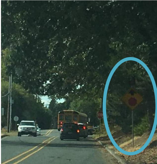
Sign partially blocked by vegetation
