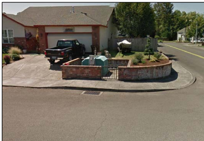
FIGURE 2.3.9 TAURUS PUMP STATION
