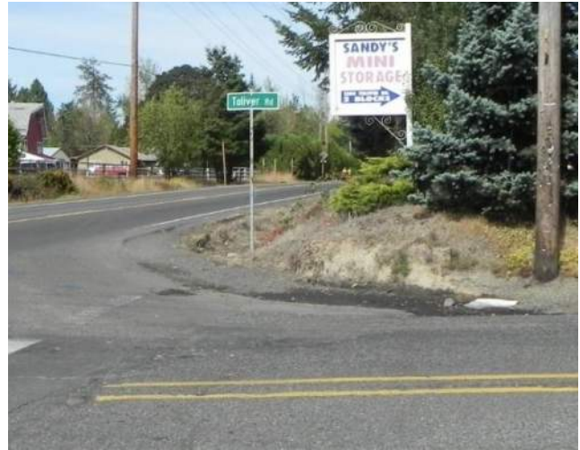
View from east leg of Toliver Road, looking north
