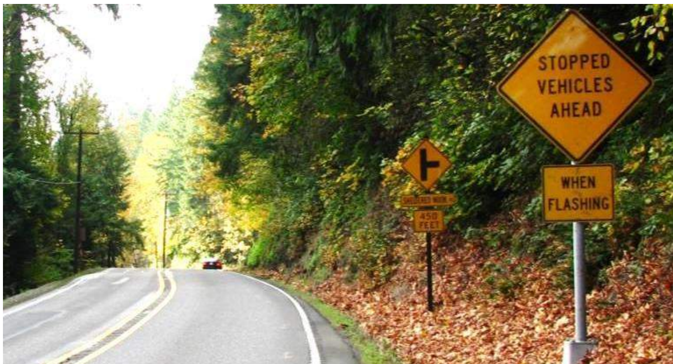
Example of actuated queue warning system on Cornelius Pass Road
