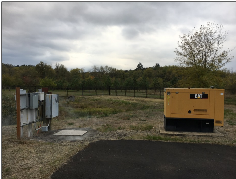
FIGURE 2.3.6 STOWERS PUMP STATION
