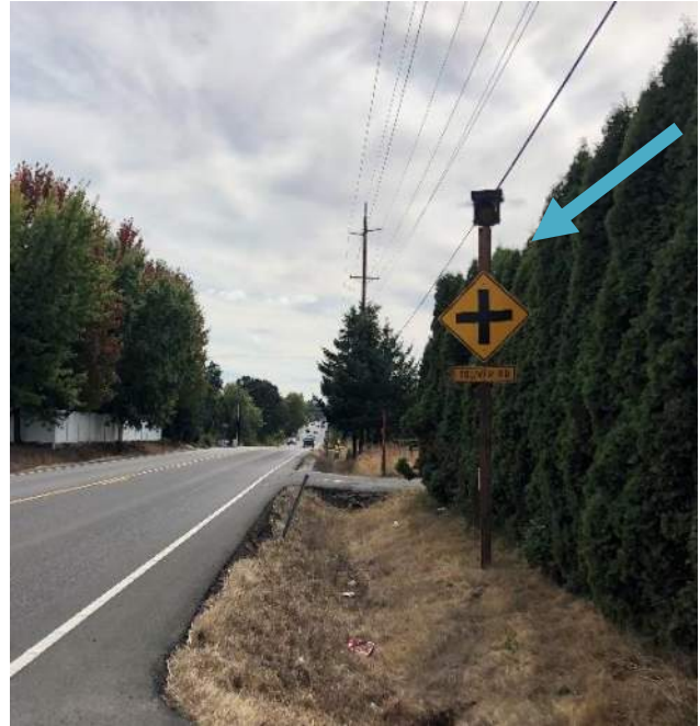
Advanced warning sign with gap between flashing beacon and sign
