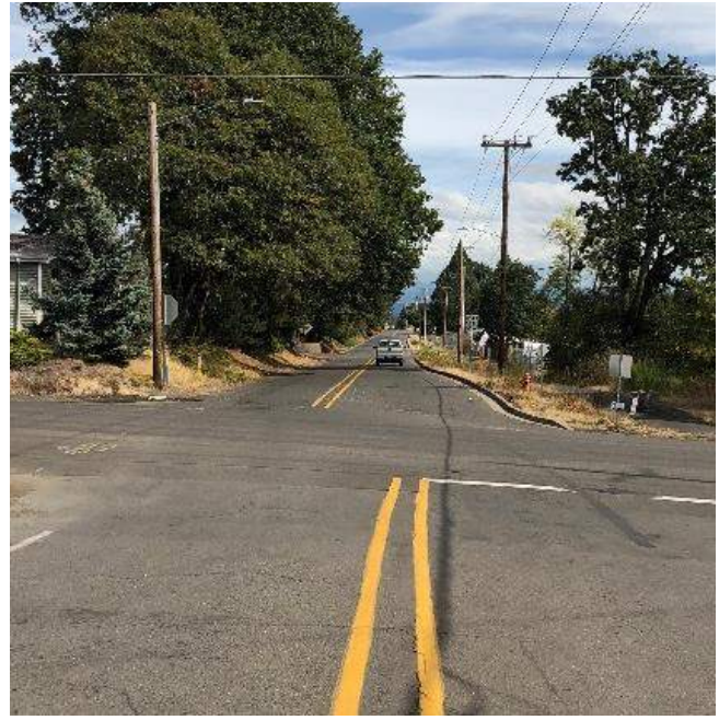
View looking east from the west leg of the intersection (Toliver Road) illustrating the intersection offset
