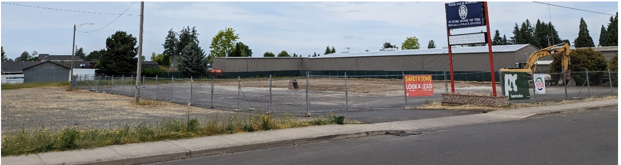
Figure 1- Site today, old bowling alley demolished and ready for new construction
