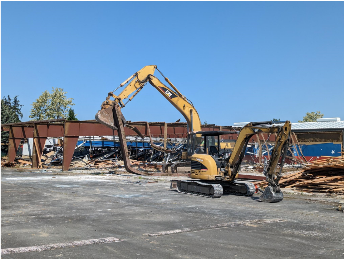
Figure 4- Bowling alley demolition
