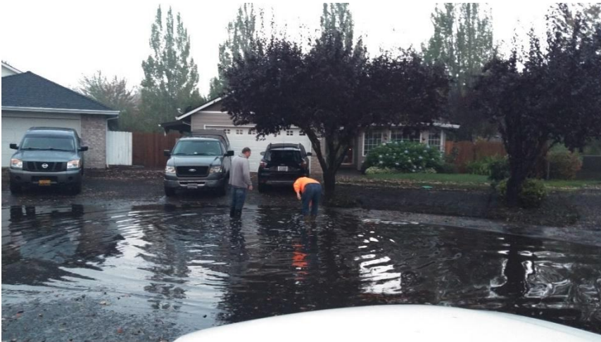
Wildfire ash mixed with tree leaves to form a paste that clogged many catch basins in town, requiring crew response to clear (Left).
