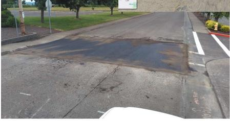
Nothing is going to solve this kind of road breakup but a full dig out. When hot patches are done today, like for the new crosswalk shown here, the City installs 6-12 inches compacted base rock over a layer of geo fabric, and at least 6 inches of asphalt. Below: the new crosswalk turned out well, but budget only allows Molalla to perform a few such digouts each year. More reporting on streets will be coming next month.
