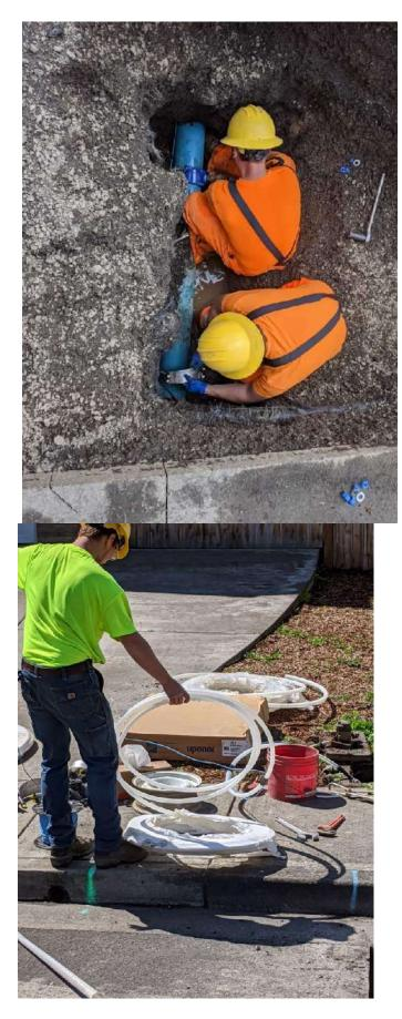
City Crews are constantly replacing and repairing water services and mains. Left, two new service saddles are placed on an 8" PVC pipe in Big Meadow, replacing more corroding copper services. Below, Devin unwinds new PEX Pipe for these new services, and Rich tightens steel bands on an older leaking mainline in July.
