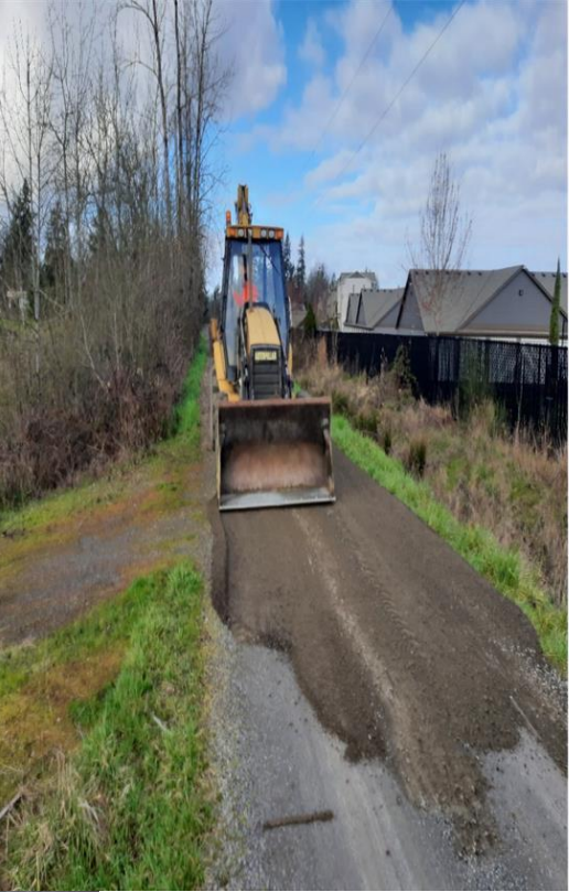
Utility Crew flushing dead end water mains (left).
