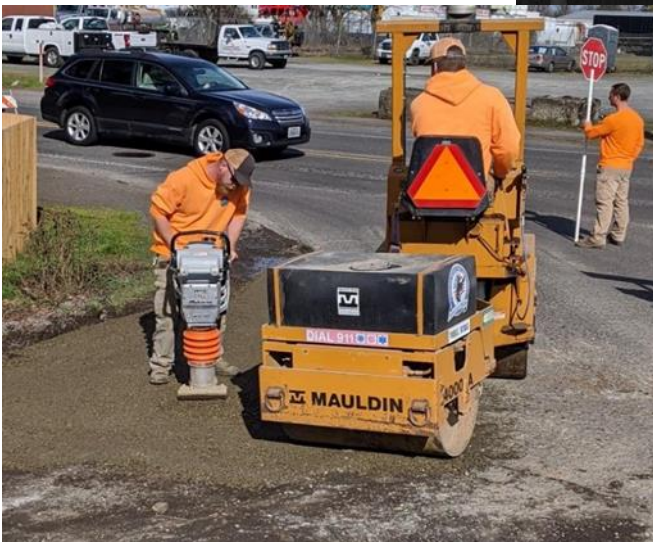
Shaver & Hwy 211 Utility Crew Preps Shoulder for Asphalt
