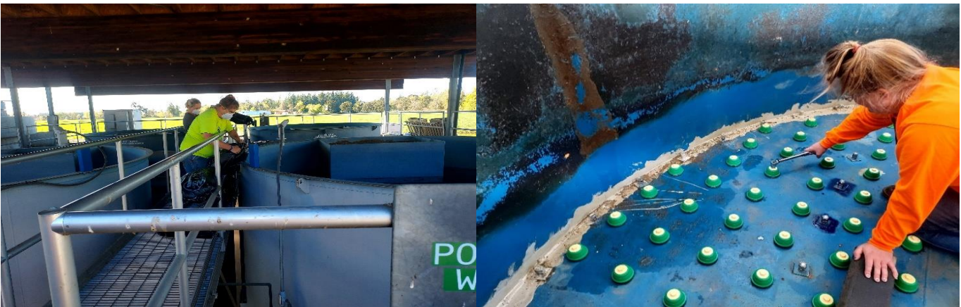
Molalla WWTP Operators Rebuild the #4 Media Tank
