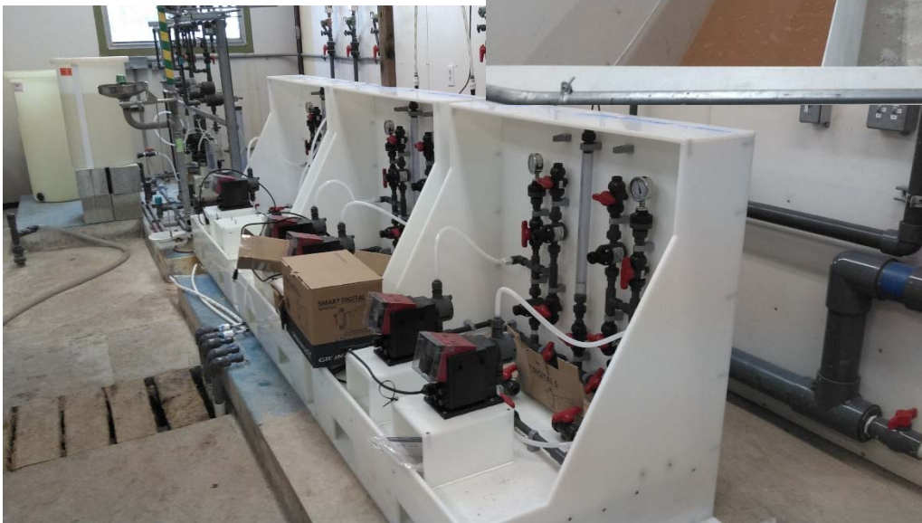
The new Chemical Feed Pumps (left) have also been installed and are schedule for testing next week (June 23 rd ).
