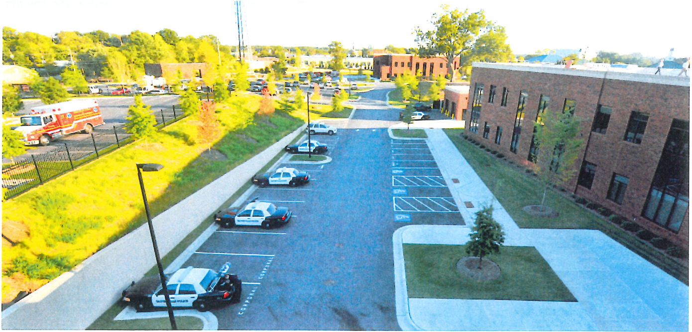
↑ CITY OF GAINESVILLE PUBLIC SAFETY CENTER, GAINESVILLE, GA | PROVIDED CONSTRUCTION MANAGEMENT SERVICES FOR NEW TWO-STORY FACILITY.
