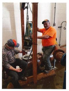
Staff at the Wastewater Treatment plant continue to make improvements, moving component by component through the plant bringing everything up to design standards. Here Operators Kevin Batridge and James Clifton replace an inline chemical mixer.
