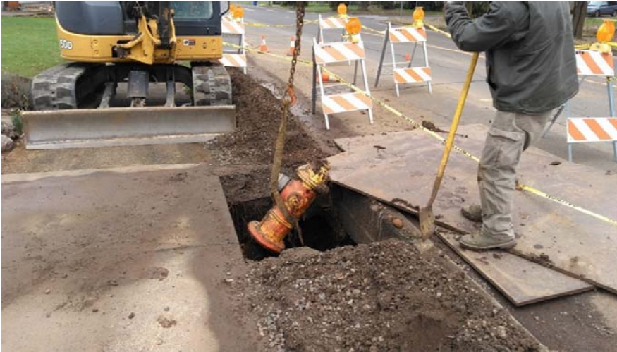
Right, Utility Crews responded to numerous water leaks throughout the two-month period. Crews replace an average of 2 services per week. Aging service lines and corroding copper lines continue to be a problem for City Crews, and the issue is being addressed by Engineers in the upcoming Water Master Plan.
