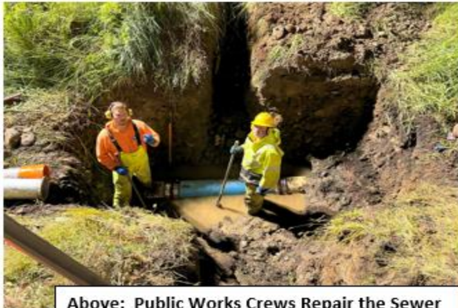
Above: Public Works Crews Repair the Sewer Main that was Damaged in the Roundabout Project.
