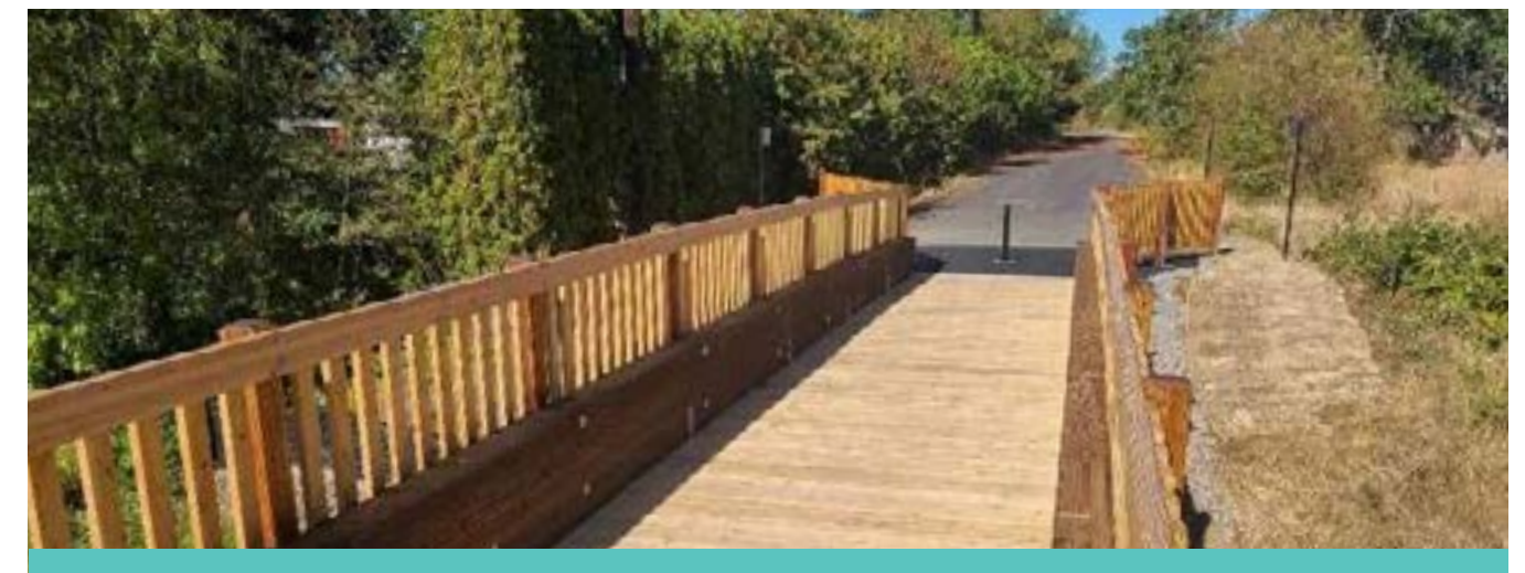
Bear Creek pedestrian bridge
