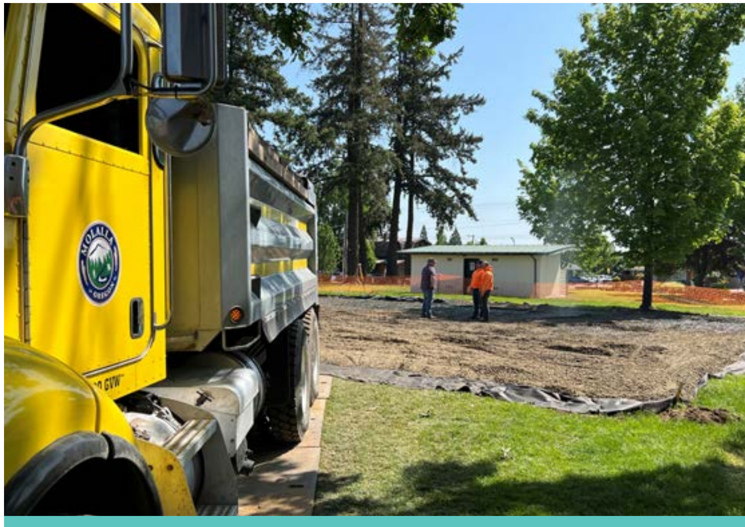
Long Park pickleball court construction
