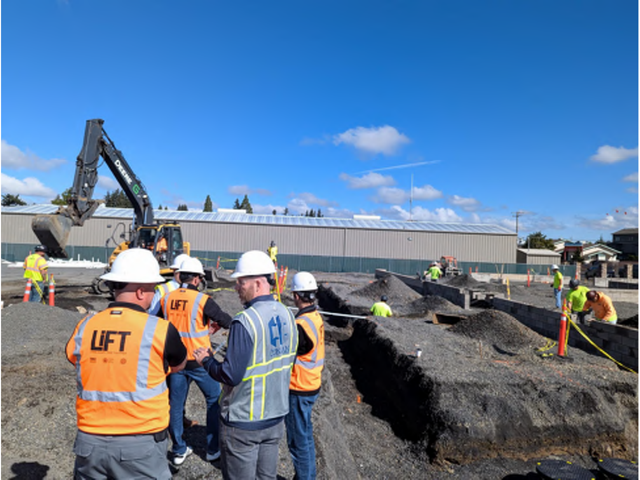
Figure 2- Project Team site walk post OAC meeting
