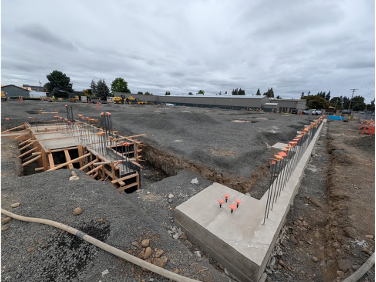
Figure 5- Building foundation footings complete
