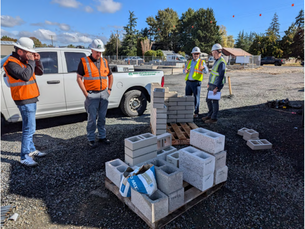
Figure 4- Team reviewing sample CMU block material
