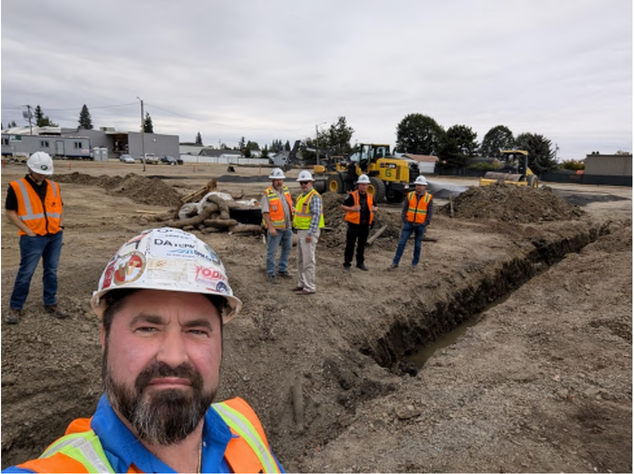
Figure 7- Team reviewing site conditions
