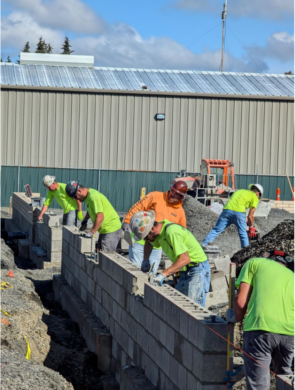
Figure 3- P&C work crew laying CMU walls
