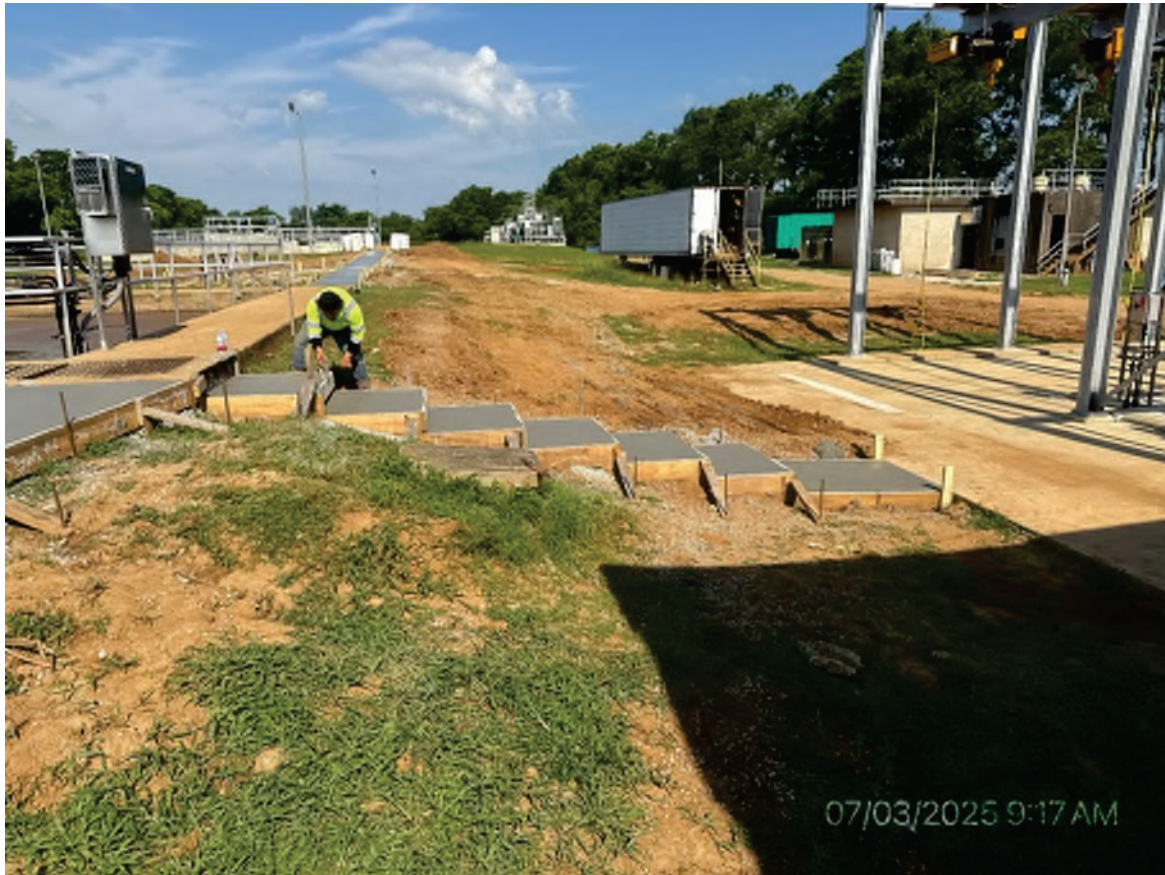
3. New Stairs Installed
