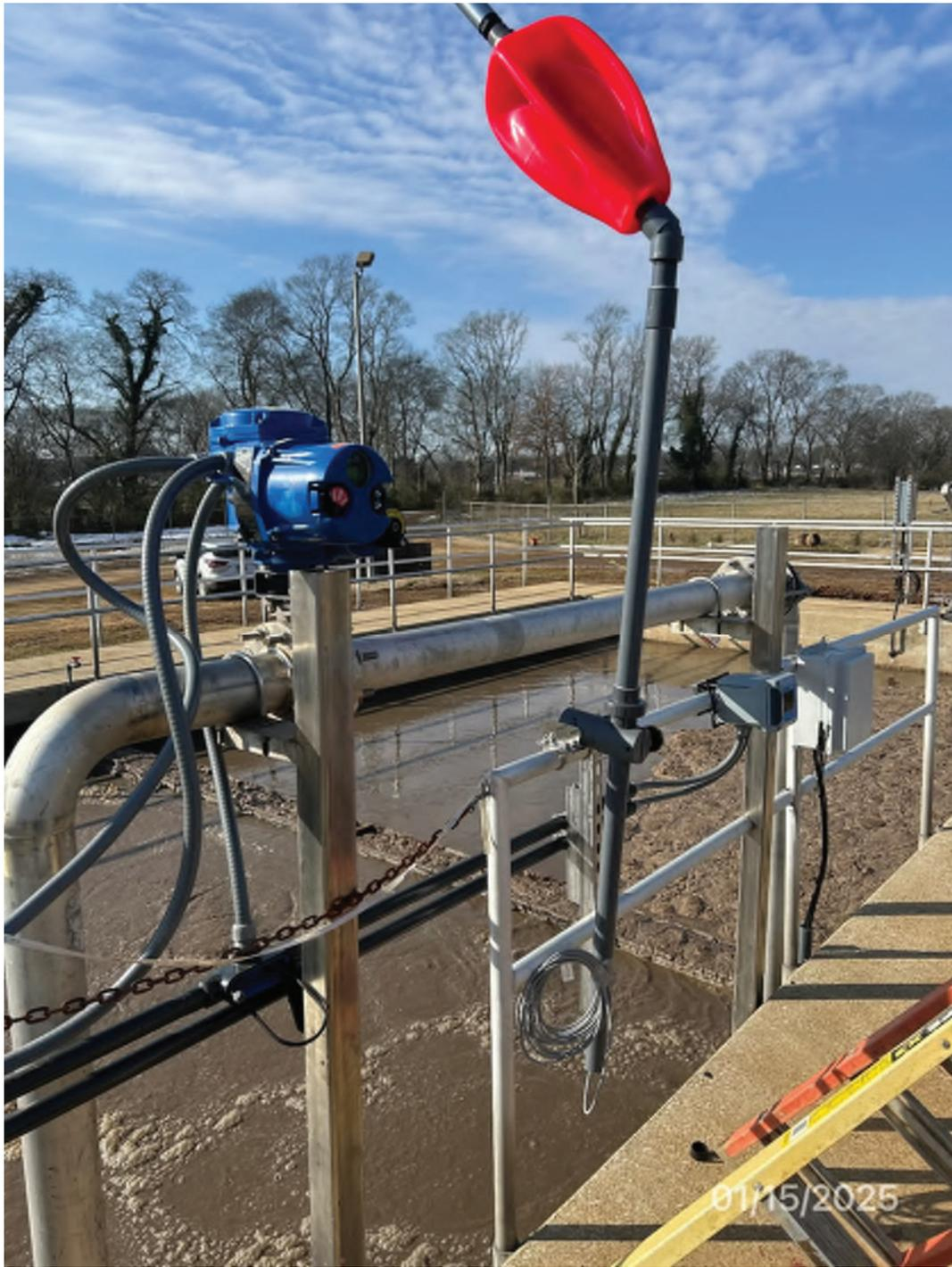
3. Treatment basin 1 with baffle wall, new air piping and control valve, and instrumentation.
