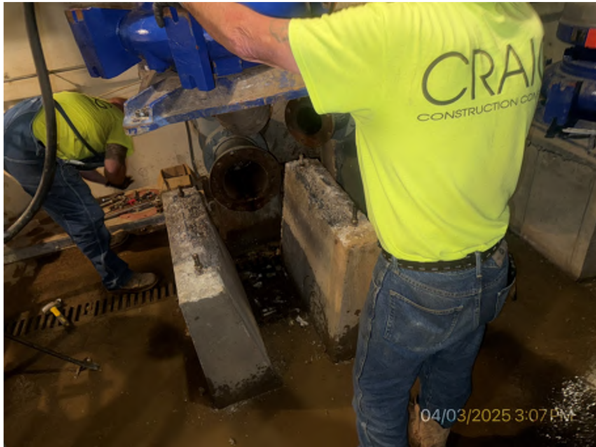
4. Installing final influent pump.
