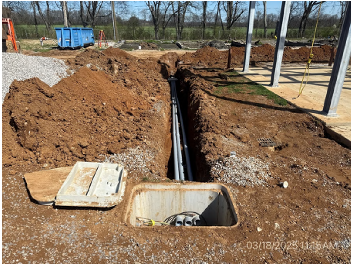
1. Conduit/Pullboxes Installed
