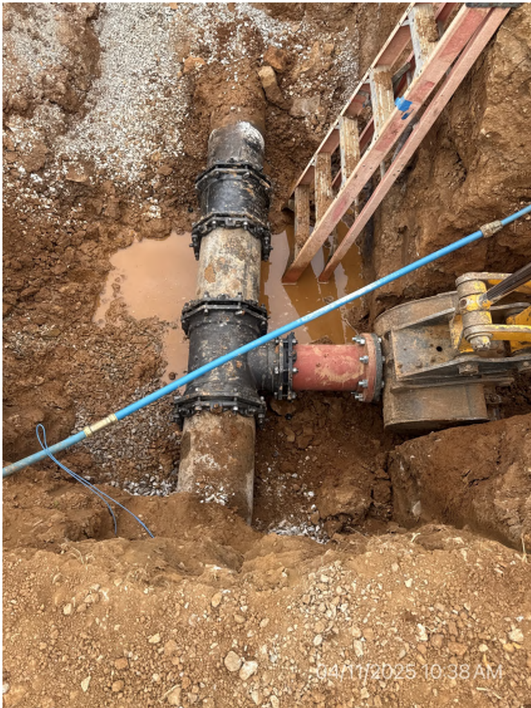
5. Installing additional piping for mixed liquor screening.
