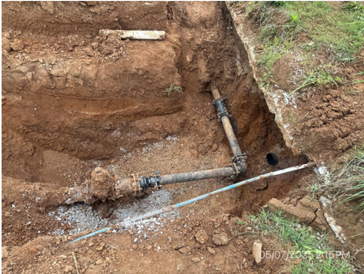
4. Installing WAS piping.
