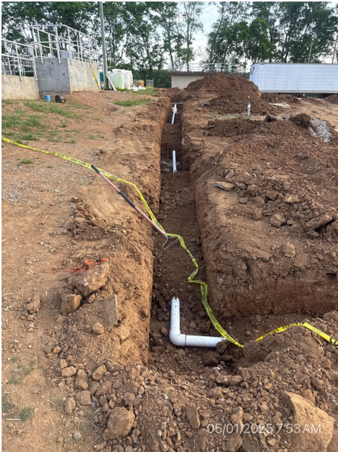
5. Installing chemical piping.
