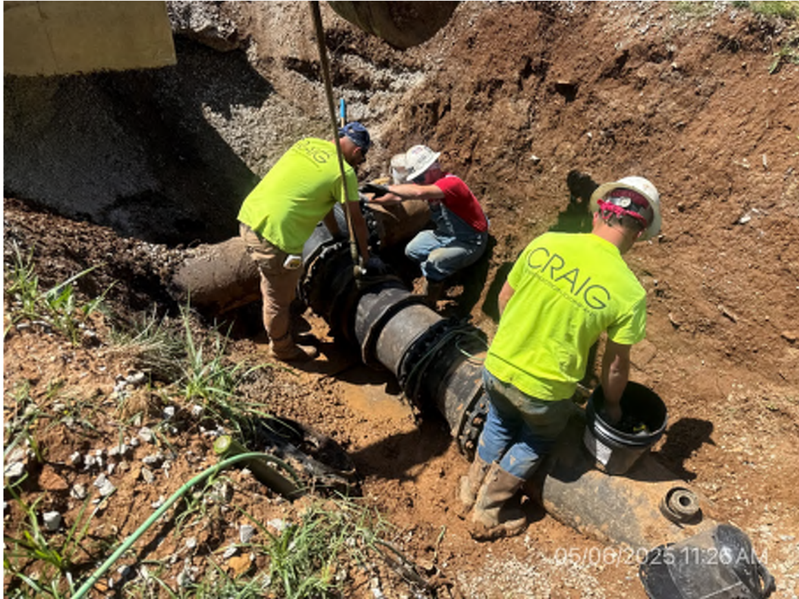
1. Installing of piping into MBR system
