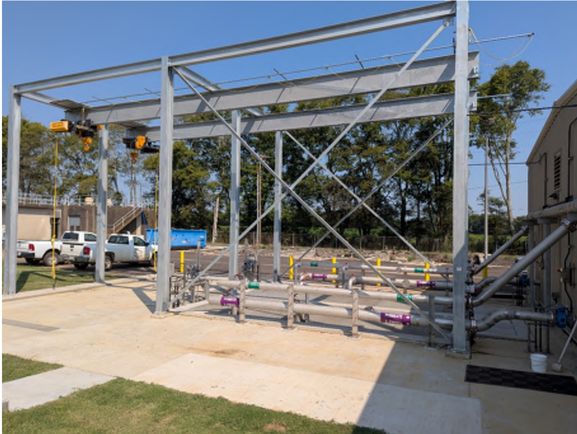
1. MBR basins with overhead hoists
