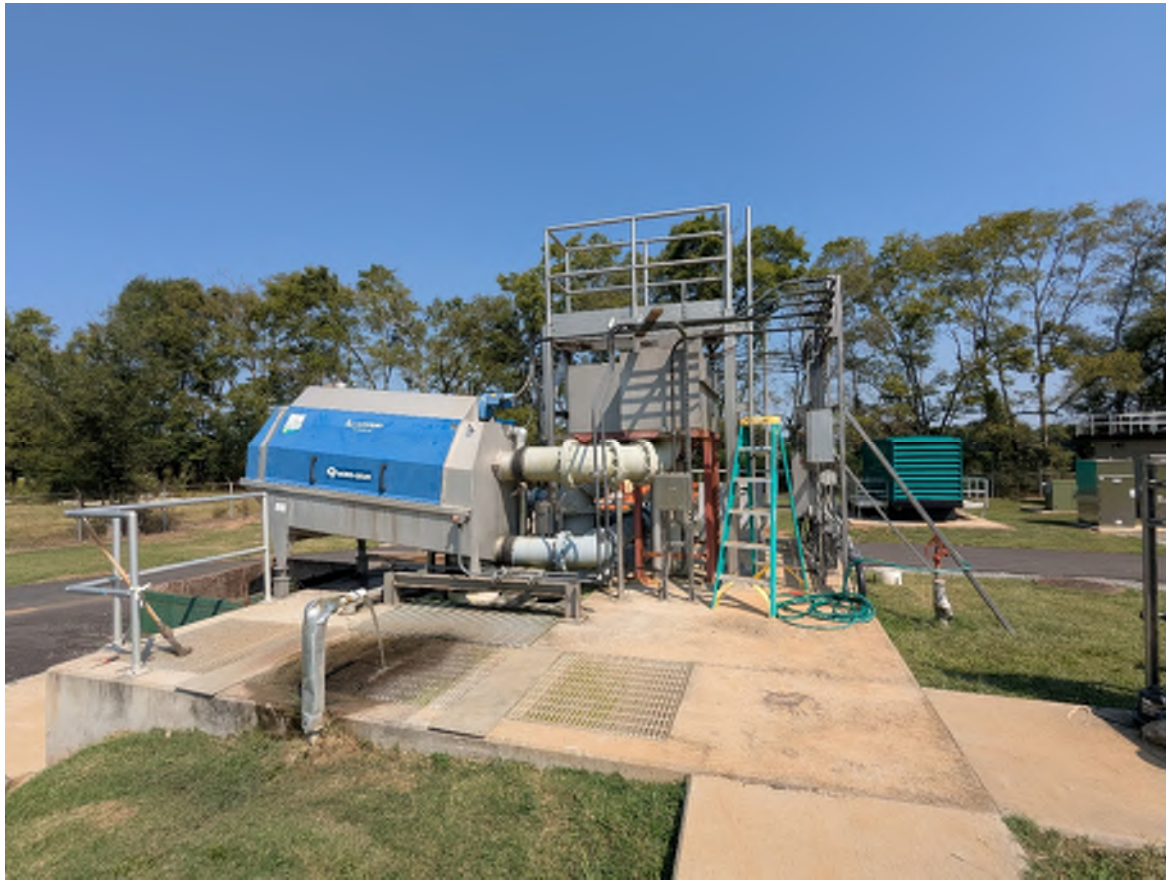
3. Headworks with fine drum screens
