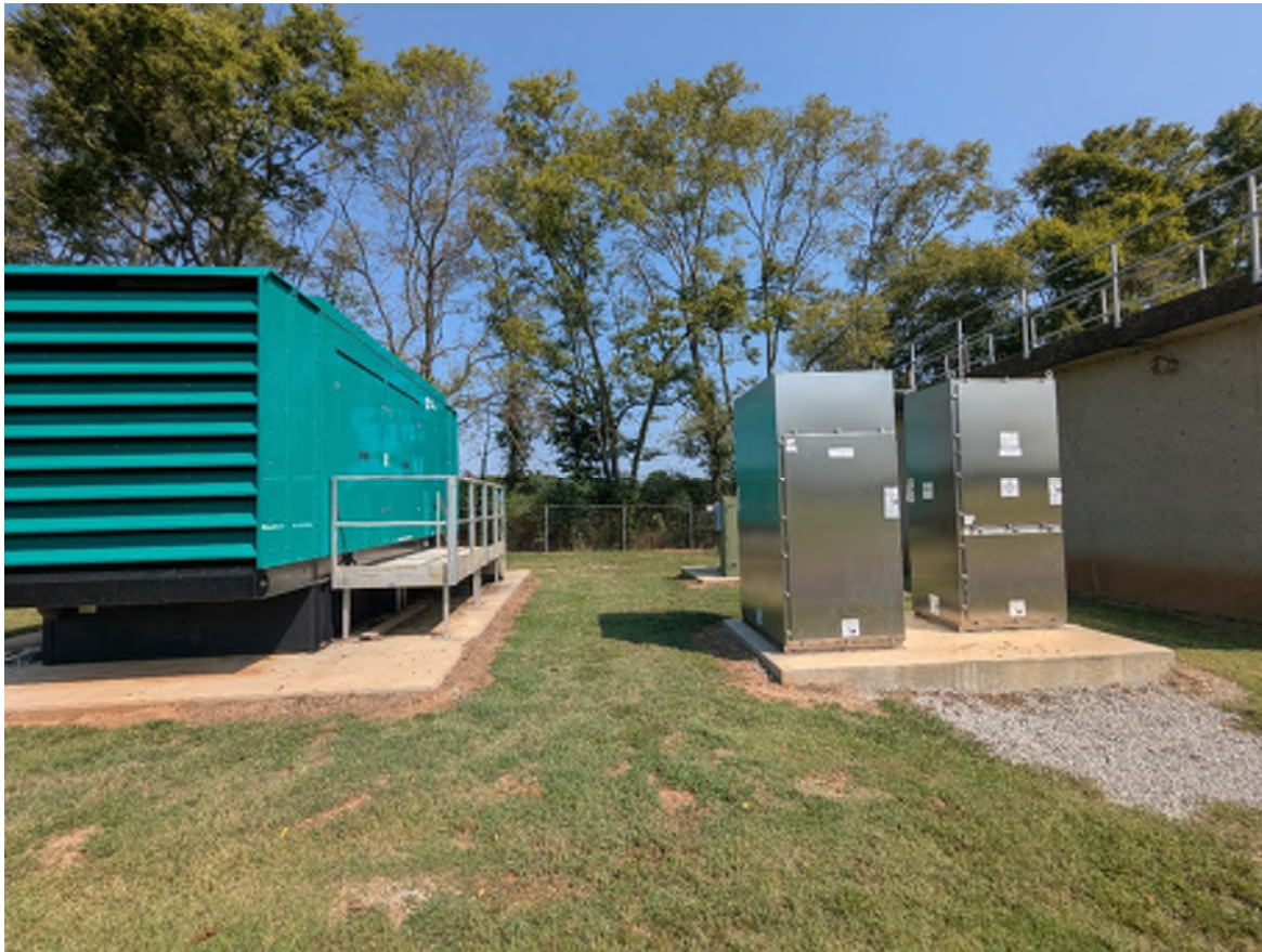
4. Generator and Automatic Transfer Switches
