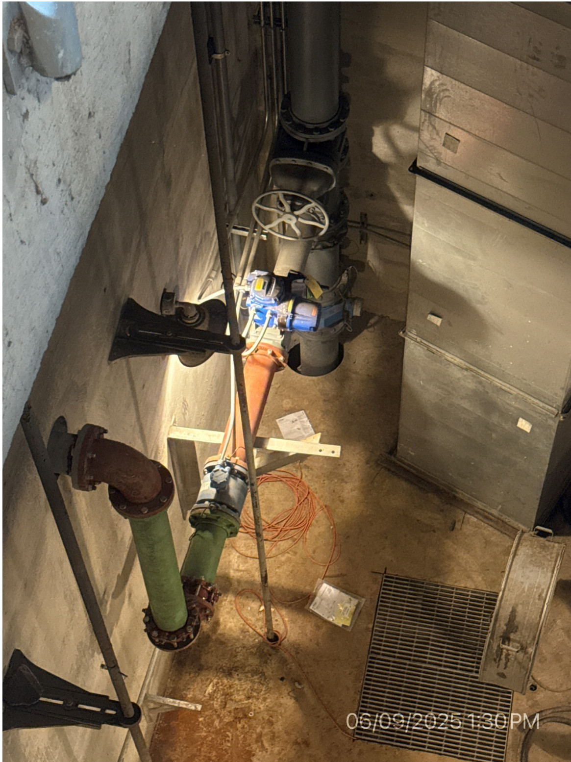
3. Installed Lagoon Return Piping
