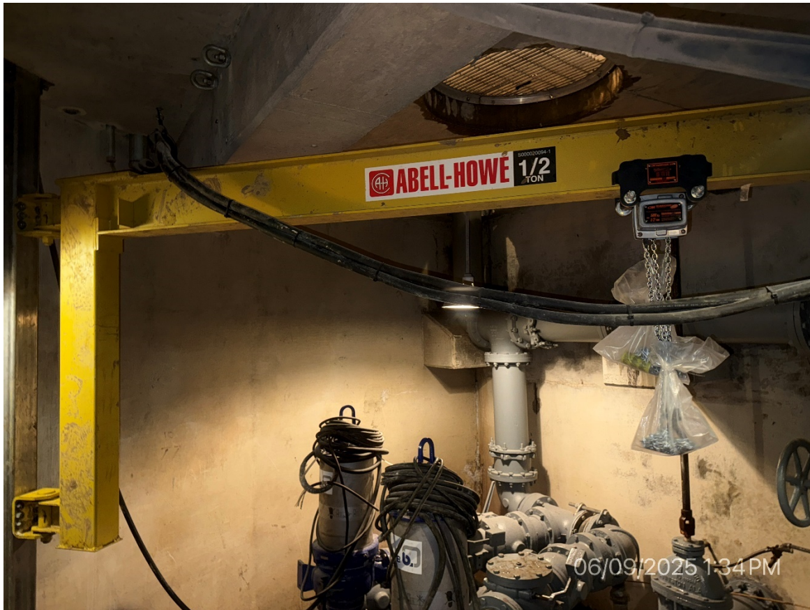
4. Installed Jib Crane at Influent Pump Station
