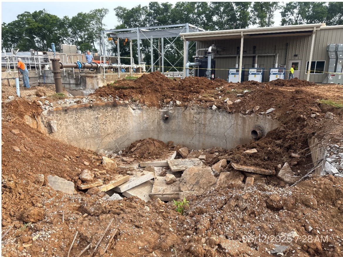
6. Demolition of Secondary Clarifier
