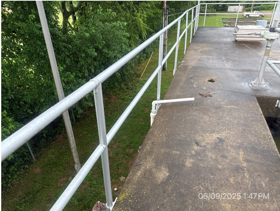
1. Repaired Handrail at Digester
