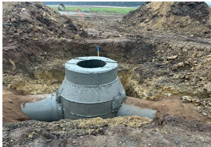
August 25, 2025 Sanitary Sewer Manhole Installation
