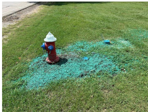
August 8, 2025 Installed Public Fire Hydrant and In Progress Site Restoration
