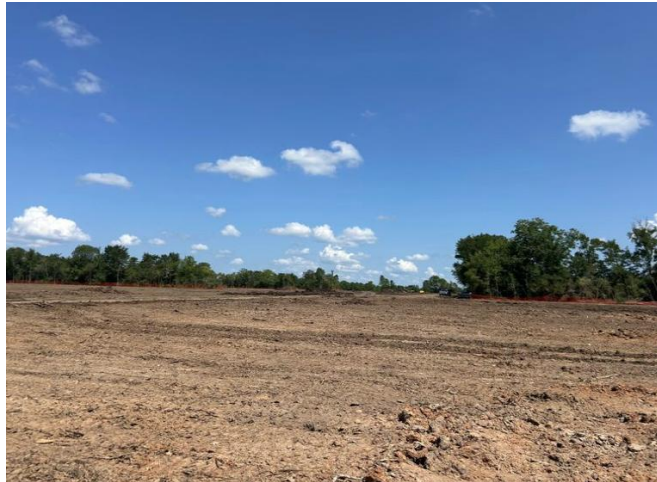
August 18, 2025 Clearing Progression
