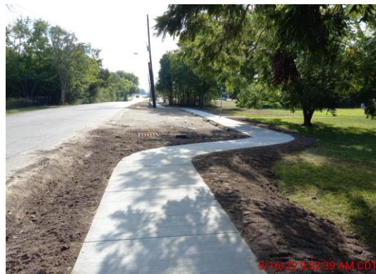
Figure 1: Newly constructed sidewalk September 16, 2022
