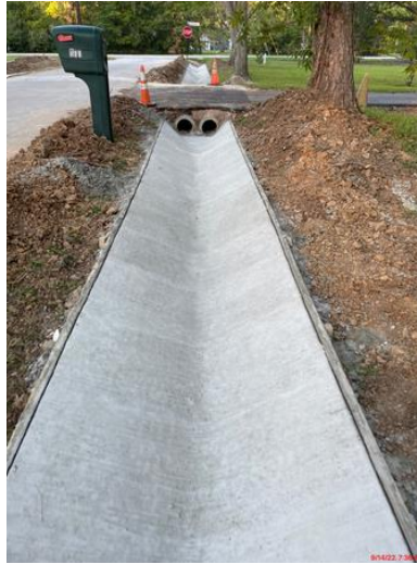
Figure 1: Newly constructed concrete lined ditch September 14, 2022
