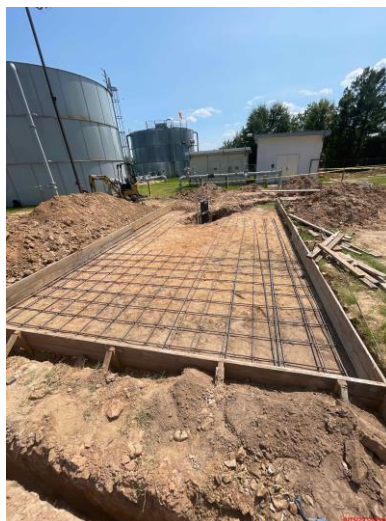
Figure 1: Generator pad formwork September 13, 2022
