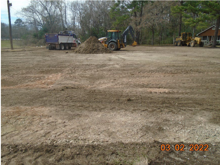
Scraping the old material from the site.
