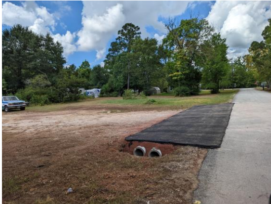
Figure 1: Culvert Replacement July 15, 2022
