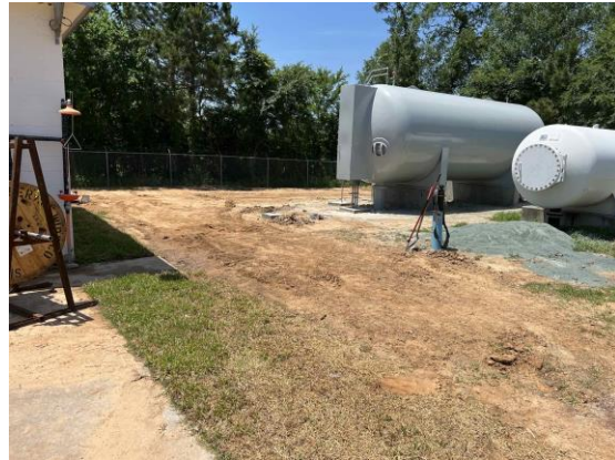
Figure 2: Hydropneumatic Tank
