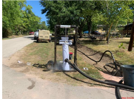
Figure 2: Sanitary Sewer CIPP Installation July 8, 2022
