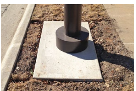
Acceptable Footer Detail
