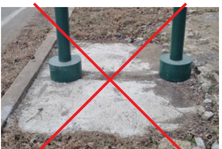
NOT Acceptable Footer Detail
