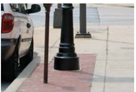
Acceptable Footer Detail
