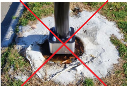
NOT Acceptable Footer Detail
