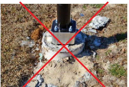
NOT Acceptable Footer Detail
