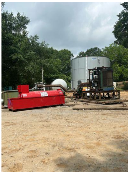
May 17, 2025 Pump for 36-hr Well Test
