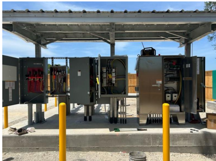
May 13, 2025 Briarley Lift Station Control Panel Installation
