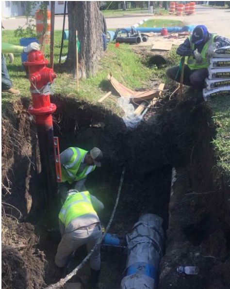
Valve Replacement on Pond St.
