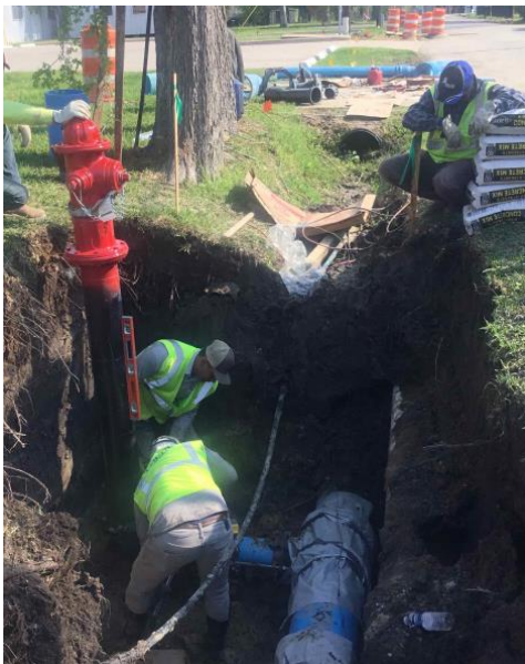
Valve Replacement on Pond St.
