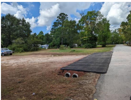
Figure 1: Culvert Replacement July 15, 2022
