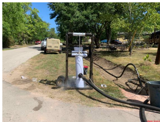
Figure 2: Sanitary Sewer CIPP Installation July 8, 2022
